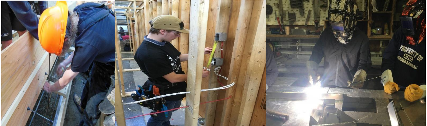
Carpentry at OC (Feb 2022)
